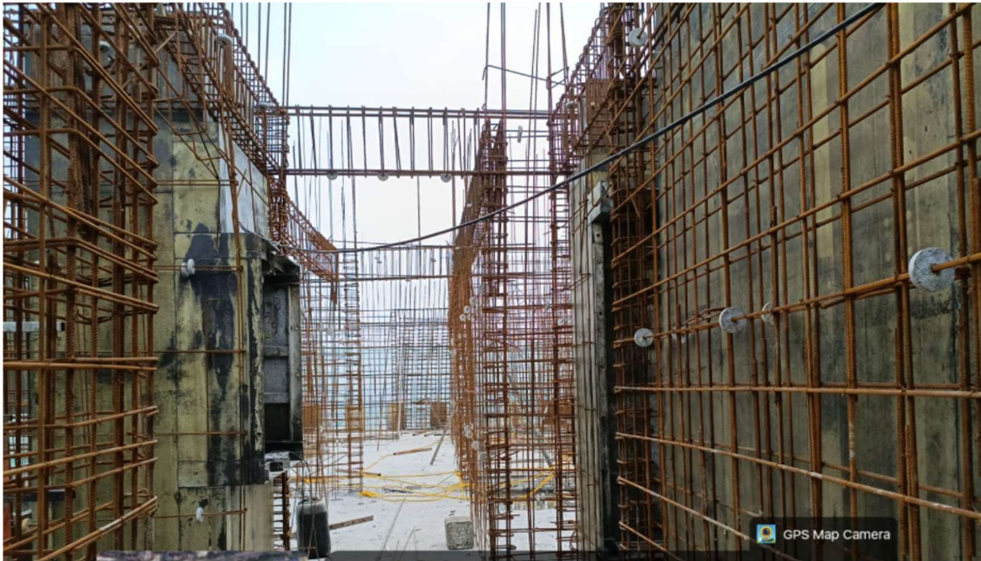
TOWER – 5's 20 TH FL. SLAB SHUTTERING & REINFORCEMENT WORK IN PROGRESS
